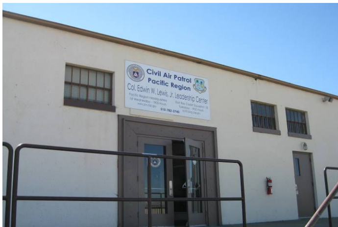
PCR HQ Building in Hayward, CA
